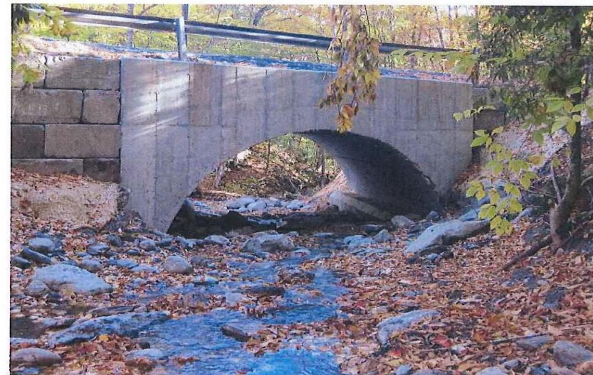
POST-CONSTRUCTION UPSTREAM END
