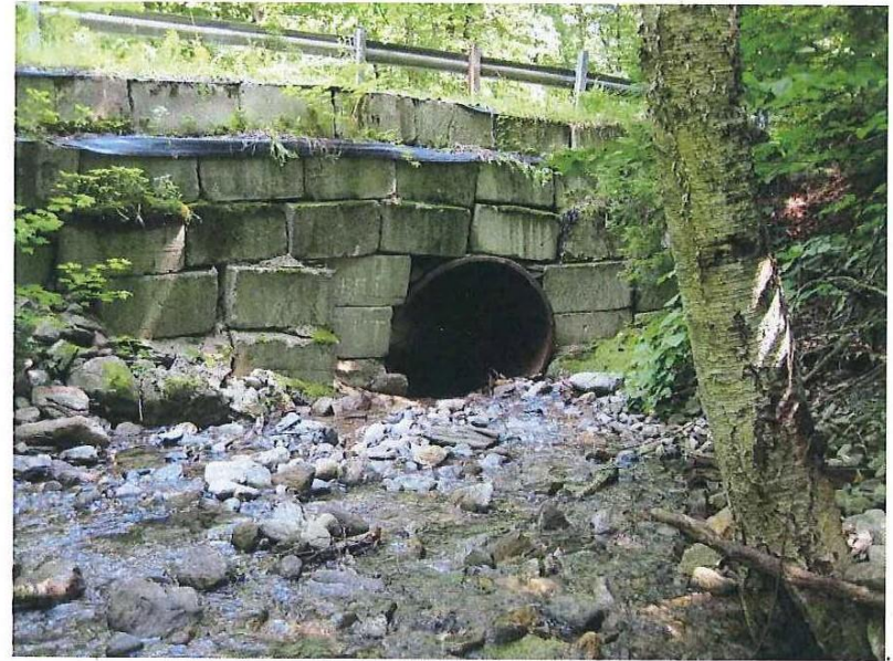
PRE-CONSTRUCTION UPSTREAM END
